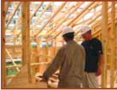
Robin Lu at a Wood-frame Construction Site in Shanghai
