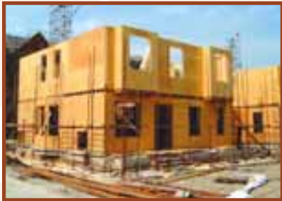
Wood-frame Construction in China
