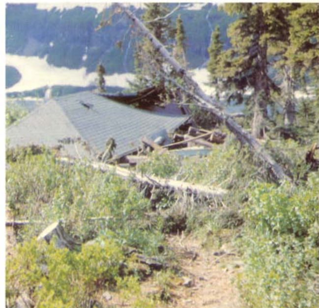
Figure 76. Damage to a picnic shelter located at the bottom of a Chute.
