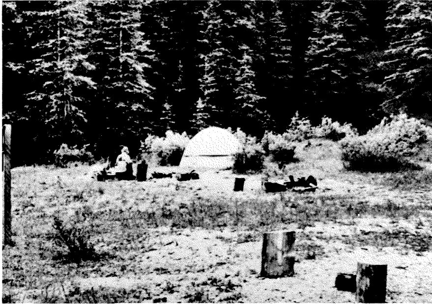
Plate 1A. View of Redearth Creek campground showing exposed soil.
