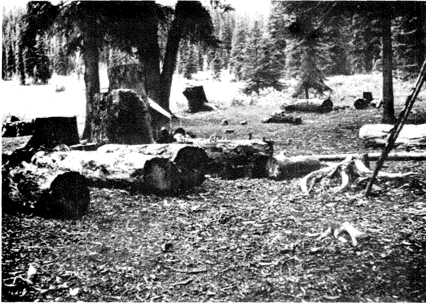
Plate 10A. Ground vegetation was completely destroyed around the wood storage and cutting place at Shadow Lake campground.
