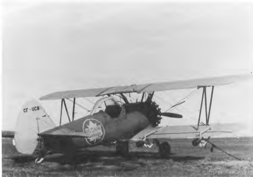
Stearman fitted with micronair emission system. Canadian Forestry Service photo.
