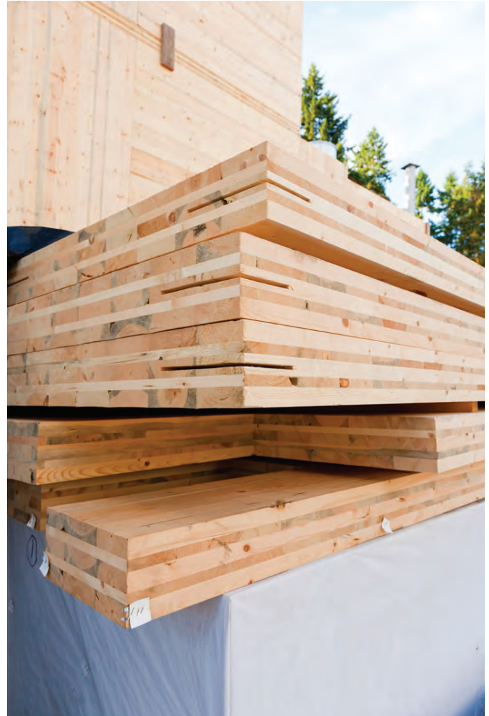
Cross-laminated timber panels.
