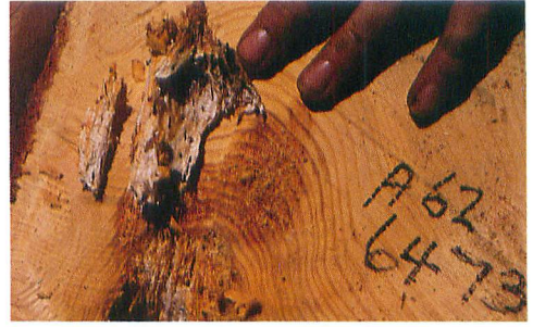
Fig. 4-28. Advanced decay caused by Poria subacida .
